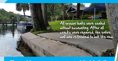
The residence owner contacted Stable Soils of Florida to inspect and provide a solution to repair their existing CMU Concrete block poured cells solid seawall on Blue Run.
