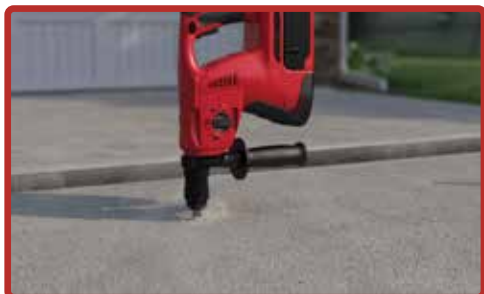
5/8" holes are drilled into the uneven concrete to allow for PolyLift ports.
